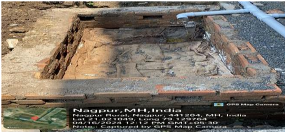
Figure 2: Constructed Magic Soak pit
